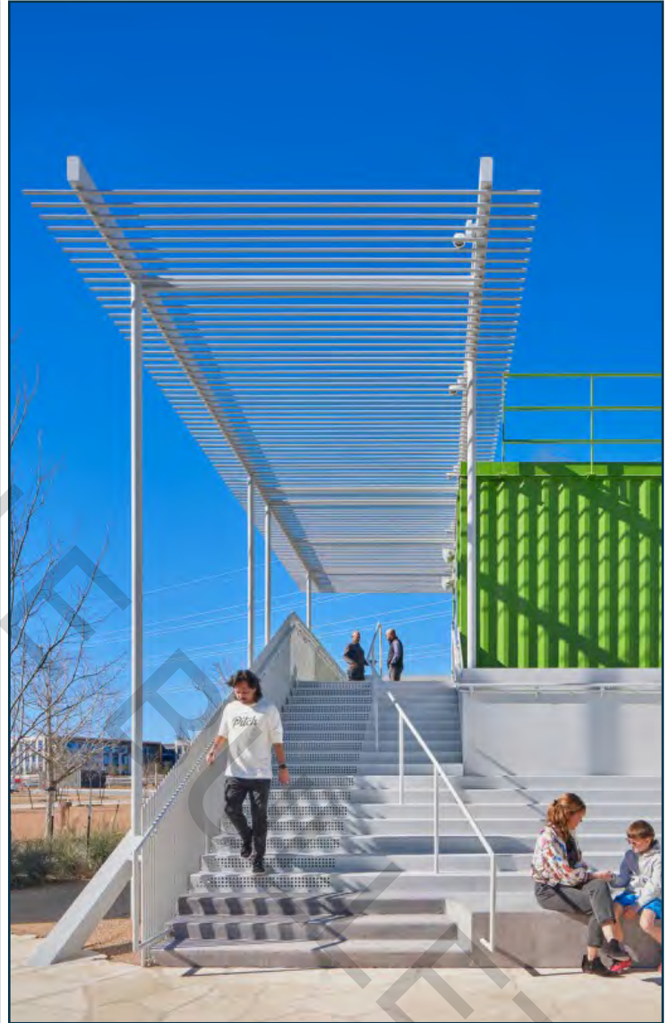
The Pitch consists of 23 shipping containers, which come in two sizes: 8 x 20 feet and 8 x 40 feet. Photo by Casey Dunn.
