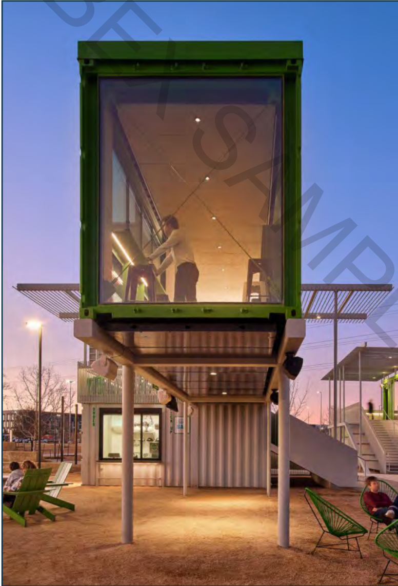
The Pitch's containers have been modified with generous glazing and staircases for access. Some have been raised above the ground with steel supports, too. Photo by Casey Dunn.
